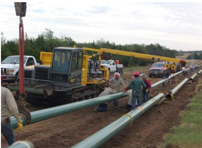
Figure 6. The Terramac's RT9 crawler carrier versatility increases when paired with welding equipment.
